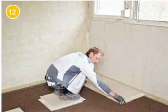
12 Now start laying the Rigidur flooring elements in the back left corner of the room. If necessary, lay out stepping surfaces made of Rigidur flooring elements to avoid stepping on the dry compound.
