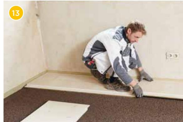
13 Lay the Rigidur flooring elements in rows longitudinally.
