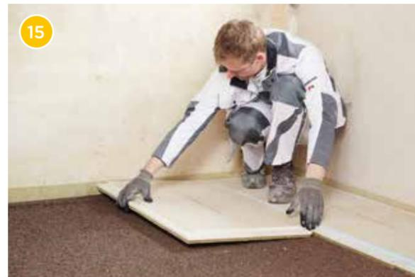
15 Now lay more Rigidur flooring elements and screw the elements in rows throughout. The transverse joints of the elements must be at least 20 cm apart.
