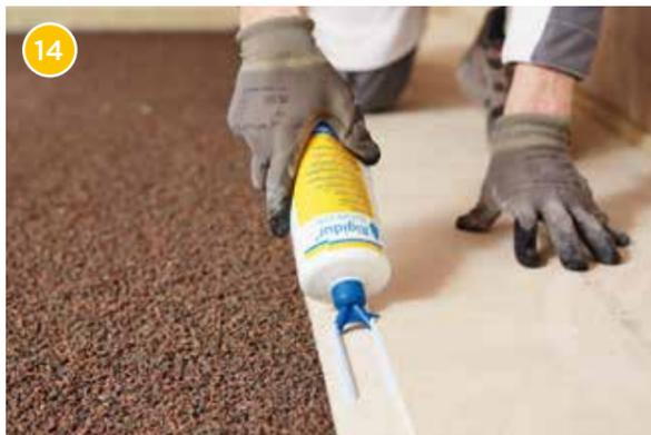
14 Apply the Rigidur Nature Line screed adhesive with the double-strand nozzle on the edge of the panel and on the rebate edges of the Rigidur flooring element.
