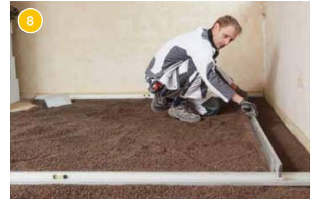
Smooth out and level the surface with a smoothing gauge over the levelling boards. Then remove the boards.
