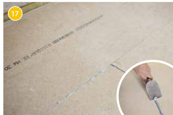
17 Residual adhesive can be scraped off along the joint to create a smooth and flat surface. The adhesive will have hardened fully after approx. 24 hours and floor coverings can be laid.
