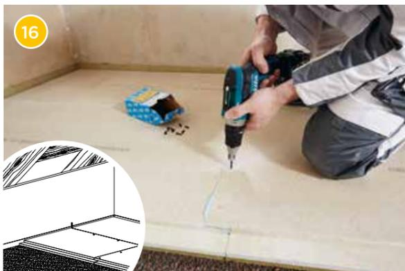
16 Connect the Rigidur flooring elements at the rebate edge with Rigidur drywall screws at intervals of approx. 25 cm.
