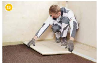
Now lay more Rigidur flooring elements and screw the elements in rows throughout. The transverse joints of the elements must be at least 20 cm apart.
