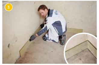
To avoid footfall sound transmission from floor to wall, lay a Rigips mineral wool edge insulation strip circumferentially. Pay particular attention to the wall corners.
