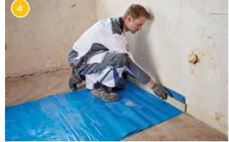
For concrete concrete floors directly bordering on the ground, lay a PE film with approx. 30 cm overlap. On wooden substrates we recommend permeable paper roll as trickle protection.
