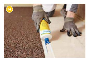
Apply the Rigidur Nature Line screed adhesive with the double-strand nozzle on the edge of the panel and on the rebate edges of the Rigidur flooring element.
