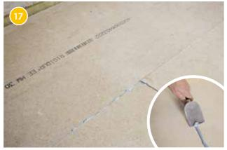
Residual adhesive can be scraped off along the joint to create a smooth and flat surface. The adhesive will have hardened fully after approx. 24 hours and floor coverings can be layed.
