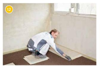
Now start laying the Rigidur flooring elements in the back left corner of the room. If necessary, lay out stepping surfaces made of Rigidur flooring elements to avoid stepping on the dry compound.
