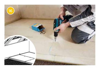
Connect the Rigidur flooring elements at the rebate edge with Rigidur drywall screws at intervals of approx. 25 cm.
