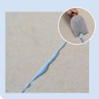
Swelling of the adhesive out of the edge area indicates optimum bonding. Once the surface of the adhesive has hardened (approx. 1 hour depending on temperature conditions), it can be scraped off to create a smooth and flat surface.
