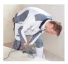
The rebate edge should be cut off where it abuts a wall
