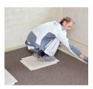
Laying the Flooring Elements on Rigidur levelling compound using "stepping stones"
