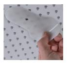
Once the Rigitone Mix has begun to harden, remove any excess carefully using the Rigips scraper and then pass the scraper back over the joints in the other direction to smooth the surface.
