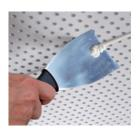
The joints and covered screw heads can be sanded after at least 24 hours. Further finishing work may be continued once the Rigitone Mix has fully dried.
