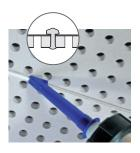
Slightly overfill the screw heads using the Rigips screw head template.
