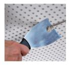
After approx. 3 hours, the joints and covered screw heads can be sanded and prepared for further finishing work.
