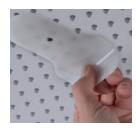
After approx. 30 minutes, carefully remove the slightly hardened excess joint filler using the Rigips scraper and then pass the scraper back over the joints in the other direction to smooth the surface.
