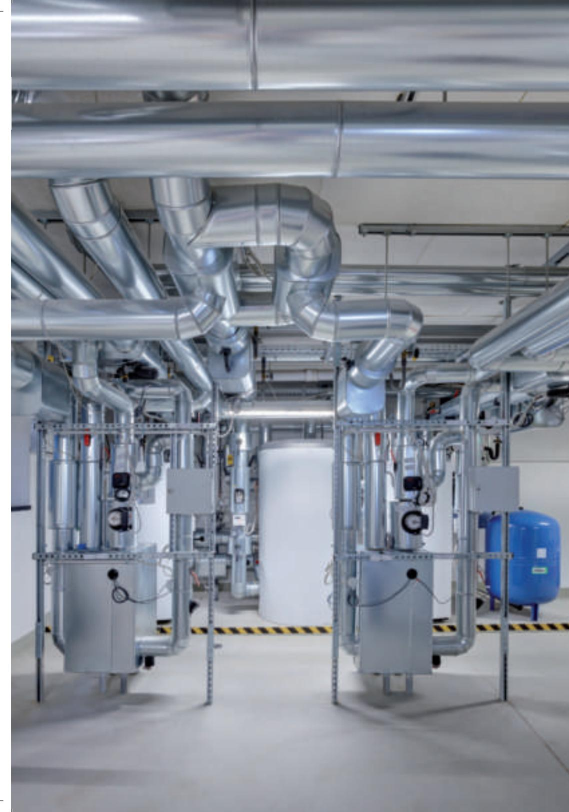
*Capillary pipe surface heating systems on ceiling and parapet areas serve to heat the rooms. By doing so, the flow temperature for the heating system can be dropped to 37°C. Heat generation takes place via heat pumps by utilising geothermal heat. Two heat pumps are installed in the main building, each with a thermal output of 33 kW.*
