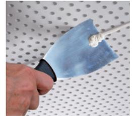
The joints and covered screw heads can be sanded after at least 24 hours. Further finishing work may be continued once the Rigitone Mix has fully dried.
